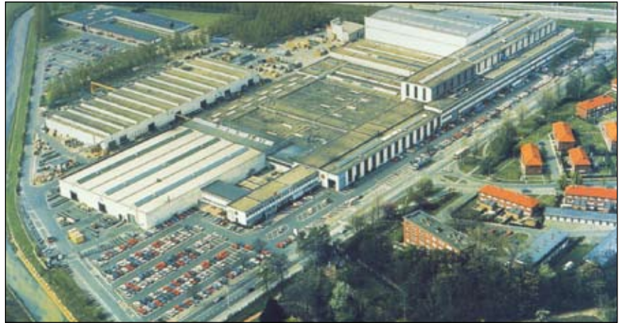
Crompton Greaves Power Systems Transformer Plant, Belgium
