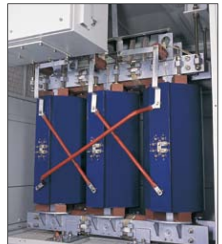
Cast Resin Transformer
