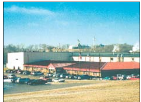
Distribution Transformer Plant Missouri, Washington, USA
