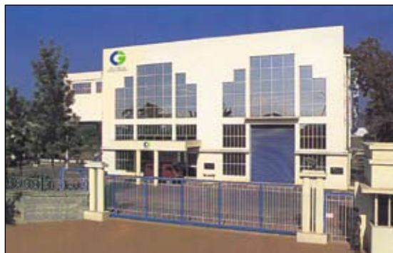
Bhopal Plant - Distribution Transformers
